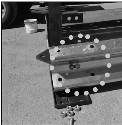
2 Bolts into End Frame
