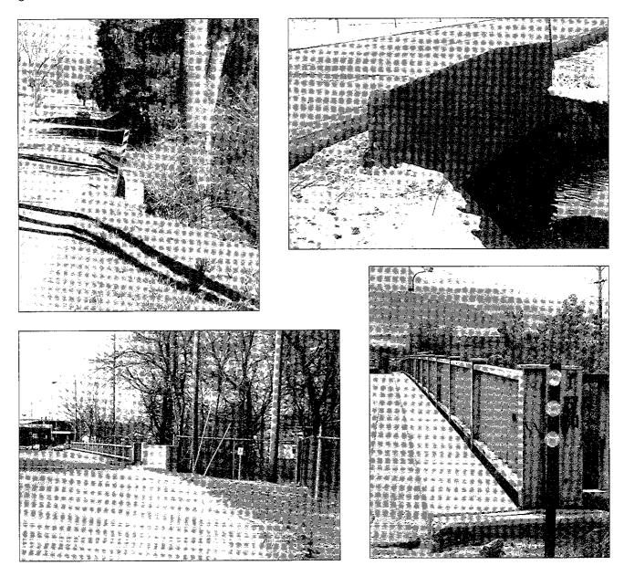
Each of these examples above are considered extremely hazardous because there is no approach guardrail on any of these rigid bridge rail terminals.
