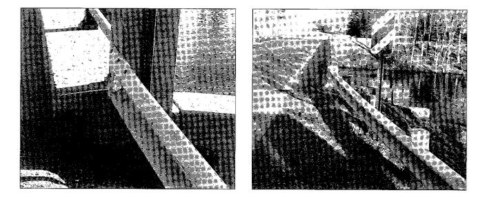
These pictures show examples of potentially hazardous approach guardrail systems. Neither of these approach guardrails is sufficiently strong enough to prevent it from deflecting, pocketing, or causing excessive force to rip or separate at the guardrail connections,
