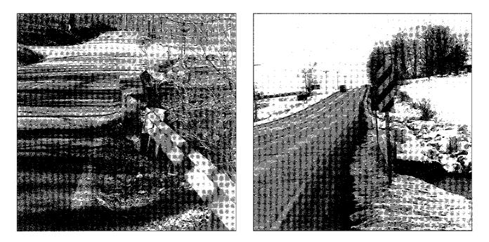
The photo at the left is an example of a bridge rail/culvert head wall that a driver might not see at night or in rainy weather. The driver could hit it, or when becoming aware of it, abruptly turn into the other lane. The photo at the right demonstrates how effective object markers can be in warning a driver of the potential hazard.
