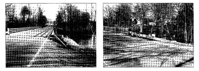
Note also the turned down ends of the guardrail present an additional potential vaulting hazard on higher-speed roads.
