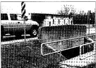
An approach guardrail must be of sufficient length to prevent a car from going around it and into the hazardous area. The pictures below show approach guardrail that is not of sufficient length (referred to as "length of need" or the length of guardrail needed to shield the motorist from the potential hazardous areas).
