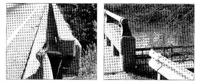
These pictures show examples of hazardous approach guardrail conditions because the guardrail is not connected to the bridge rail. Guardrail systems must be attached with the correct size and number of high strength bolts to insure they are adequately anchored.
